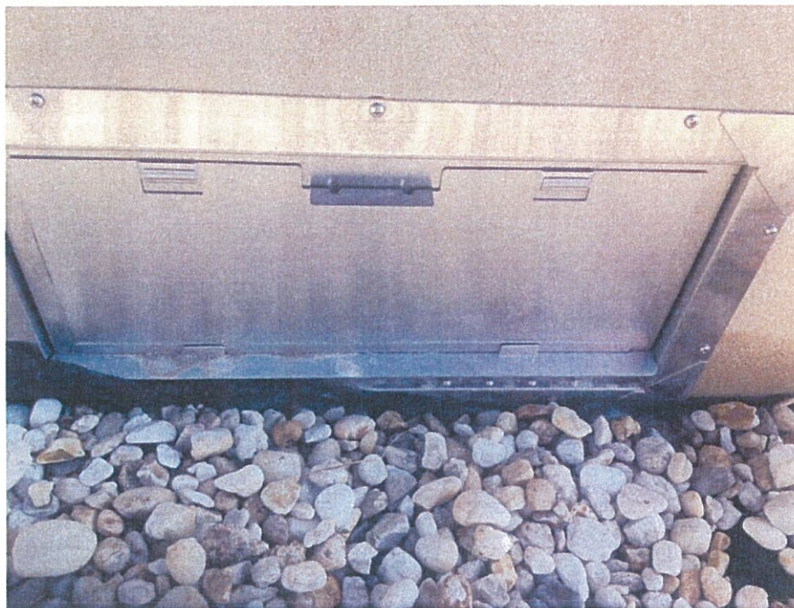
116 Demmy Avenue, Flood Vent, 04/14/13
